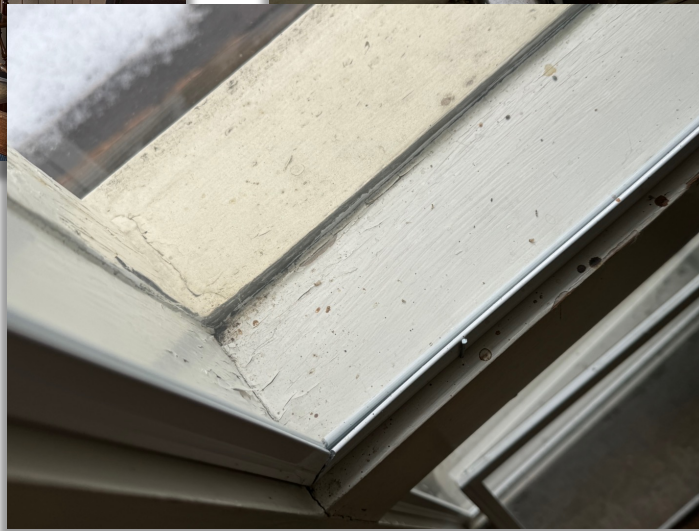
Deteriorating frames
