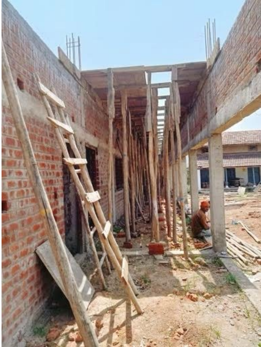
Building Porch of New Building
